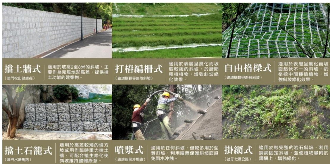
Figure 4 Six methods of reinforcing the slopes.
